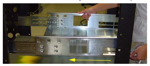
Figure 2-6: Push Shelf Unit into Rack
